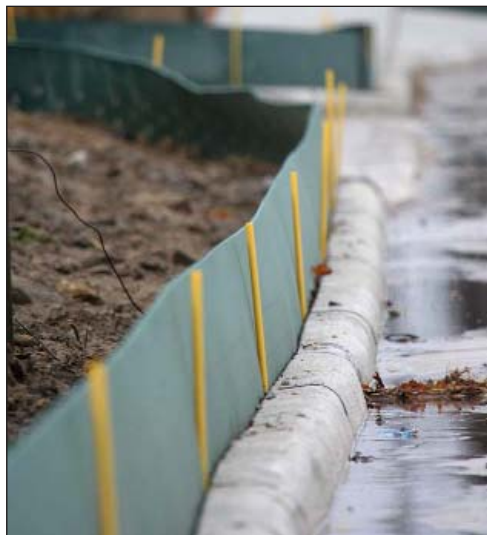
SiltShield fencing prevents storm runoff from construction sites in stormy weather.
